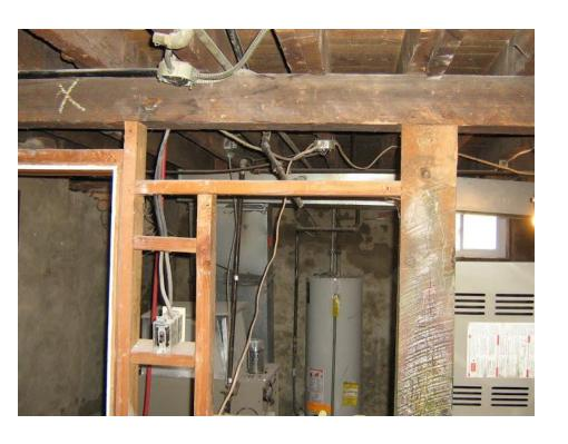
Basement mechanical room with 80% Goodman Furnace and basic water heater, both now cut in half for display in our training center.
