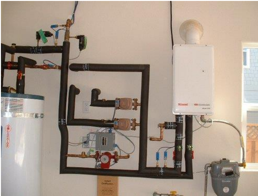
Above: SWH infrastructure installed
