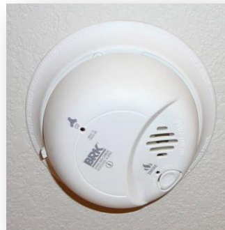
Combined CO & Smoke Alarm
