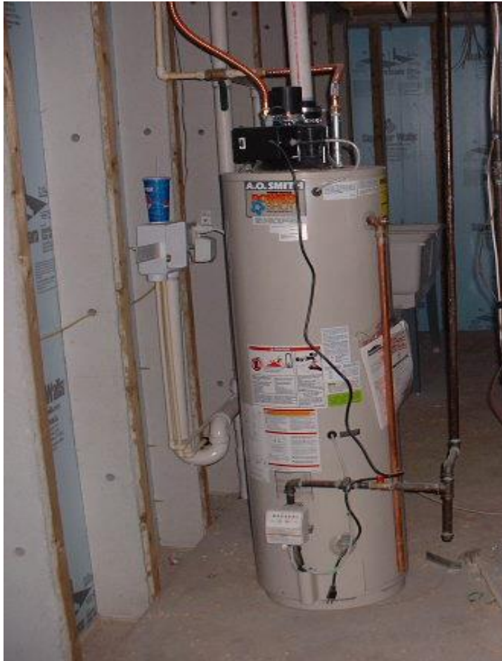
Power Vented Water Heater
