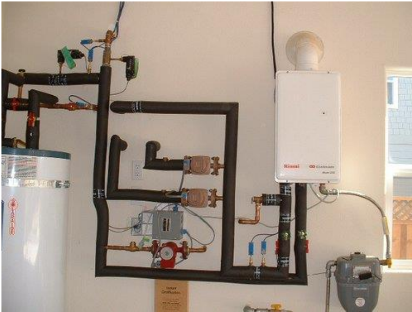
Above: SWH infrastructure installed
