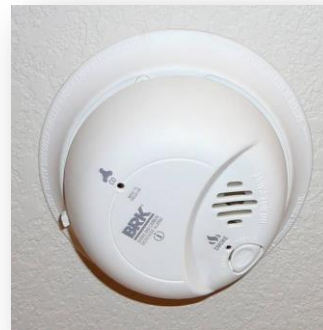
Combined CO & Smoke Alarm
