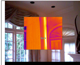
IR003087.IS2 10/8/2009 3:15:52 PM FL1: Duct/flue in exterior wall.
