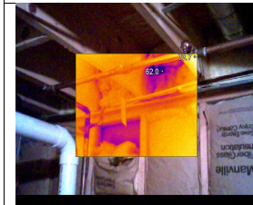
IR003094.IS2 10/8/2009 3:28:09 PM BSMT: Frame wall above foundation- air leakage at rim joist, insulation discontinuity.
