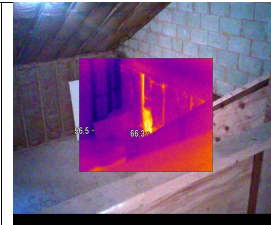
IR003092.IS2 10/8/2009 3:20:43 PM FL2: Unsealed, uninsulated ductwork in bonus room.
