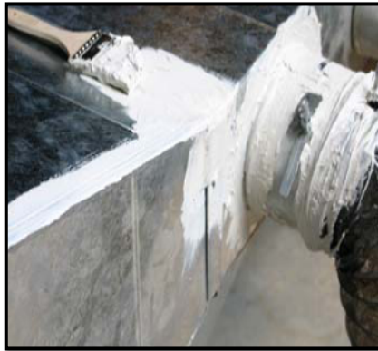
Recommended: Seal all duct connections with mastic
