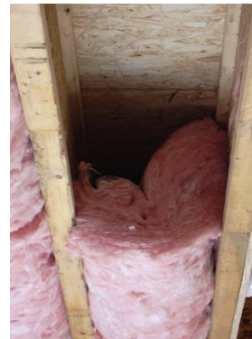
Insulation settling away from sub-floor
