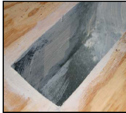
Seal the boot to subfloor/drywall connection with caulk or mastic
