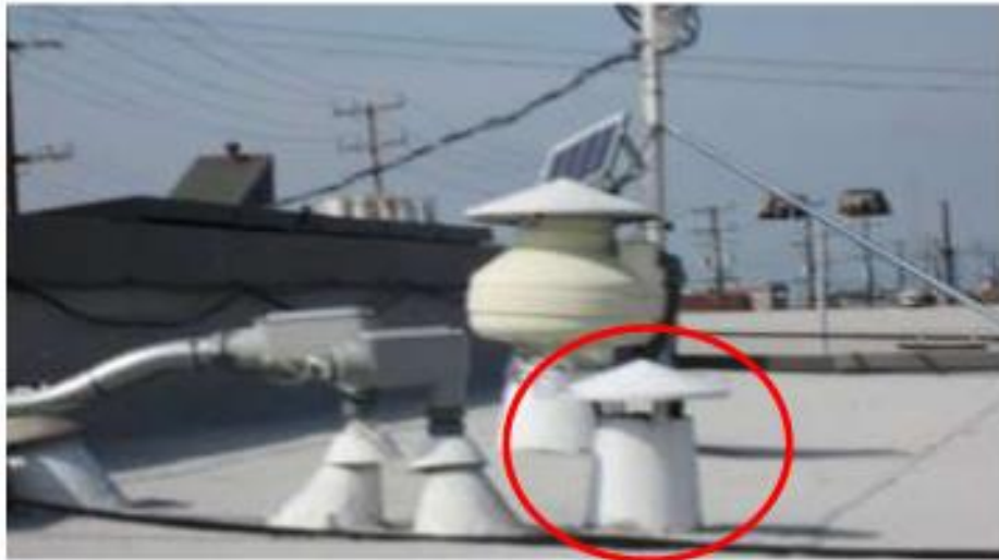
Figure 16: We located FH6's range hood outlet (circled) on its roof, but for safety reasons did not try to measure its flow
