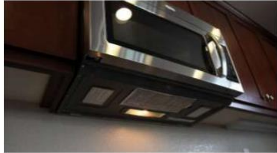
Figure 17: The dimensions and irregular surface of this typical microwave-integrated range hood in FH2 makes inlet flow measurements difficult
