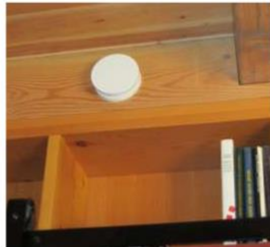
Figure 15: The ledge and uneven surface adjacent to this ERV outlet terminal made its flow difficult to measure
