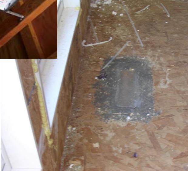
COVERING DUCT OPENINGS DURING CONSTRUCTION
