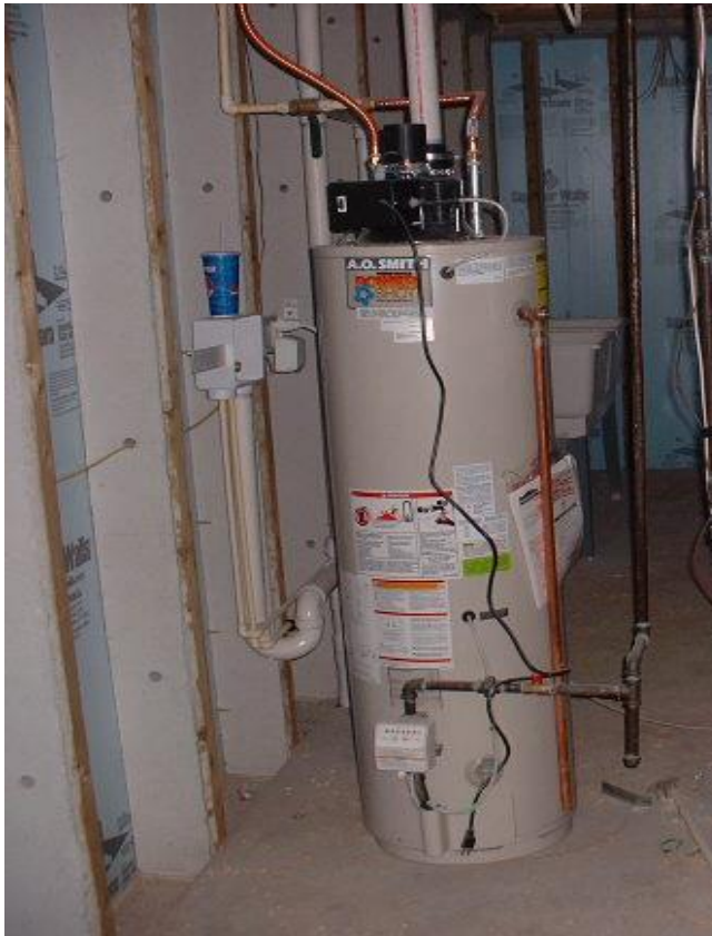
POWER VENTED WATER HEATER
