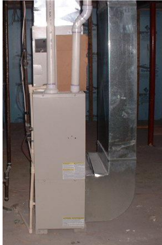
DIRECT VENTED FURNACE
