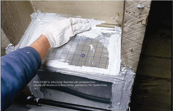
SEALING WITH MASTIC
