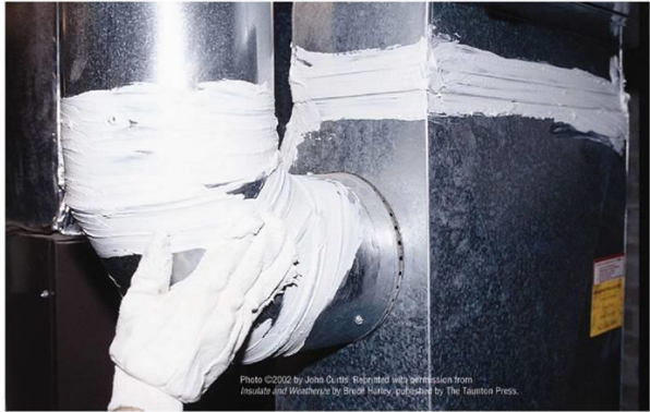
SEALING WITH MASTIC
