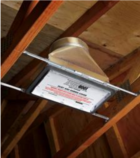
COVERING DUCT OPENINGS DURING CONSTRUCTION
