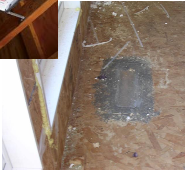
COVERING DUCT OPENINGS DURING CONSTRUCTION
