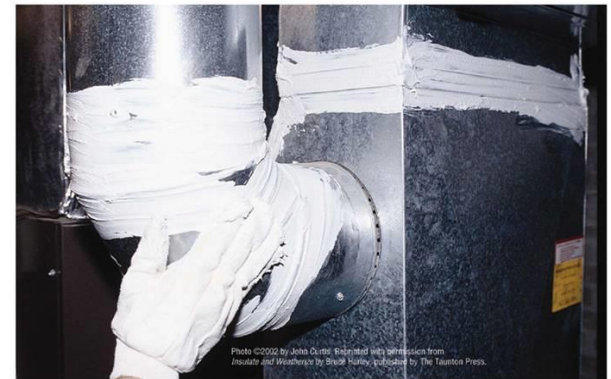
SEALING WITH MASTIC
