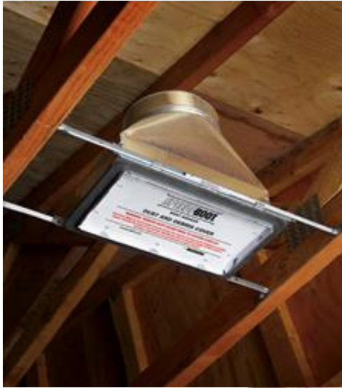
COVERING DUCT OPENINGS DURING CONSTRUCTION
