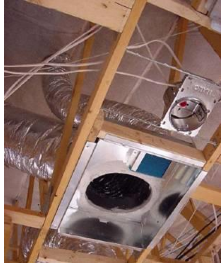
DUCTED FRESH AIR SUPPLY
