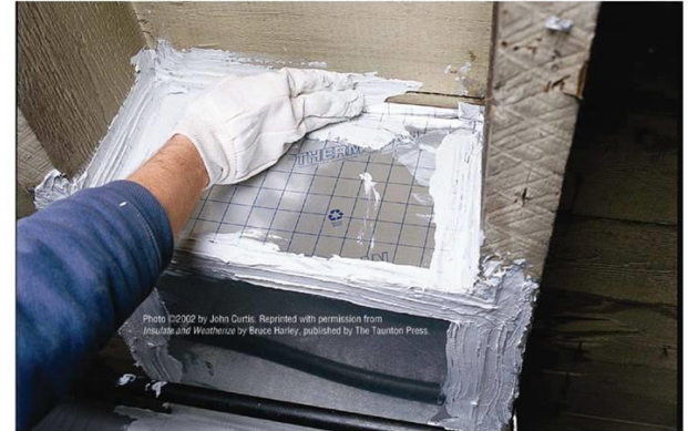
SEALING WITH MASTIC
