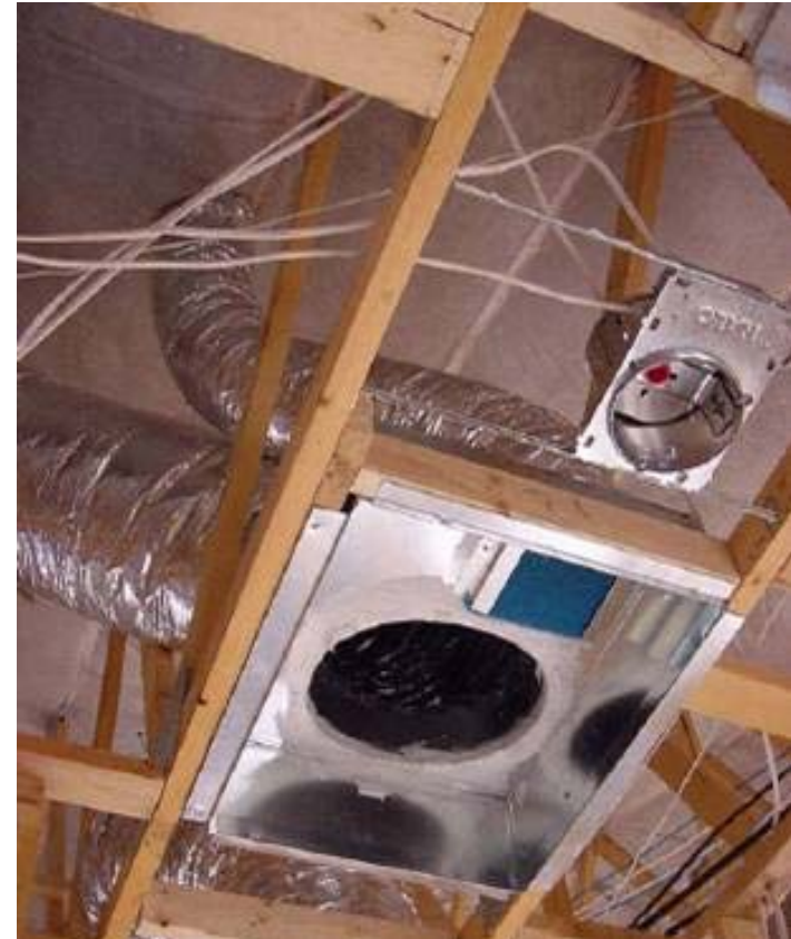
DUCTED FRESH AIR SUPPLY
