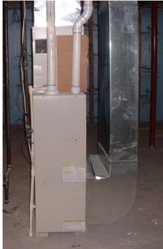
DIRECT VENTED FURNACE
