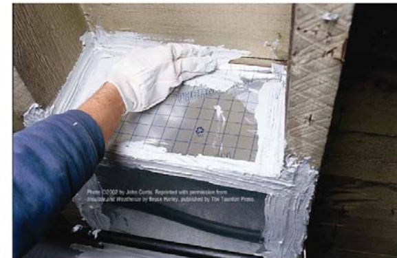
SEALING WITH MASTIC
