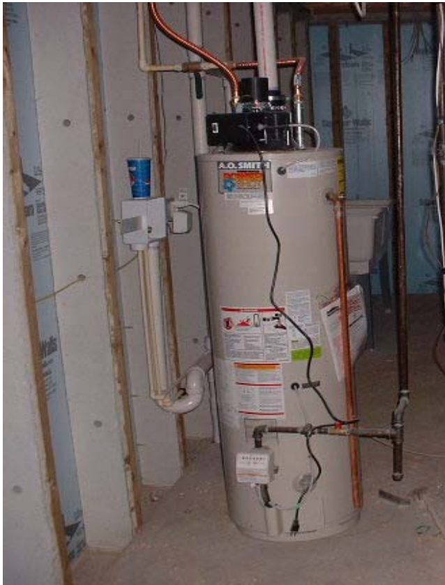
POWER VENTED WATER HEATER
