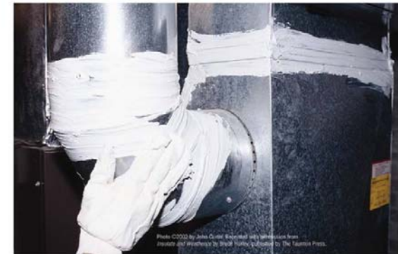
SEALING WITH MASTIC
