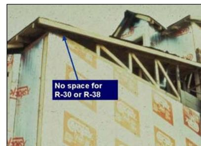
Vaulted ceilings and foam sprayed rooflines will likely need to perform a trade-off
