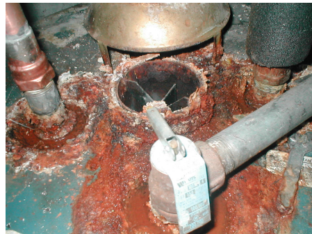
Evidence of Spillage and Improper Draft
