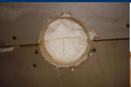
Properly sealed at panel joint
