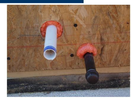
How to penetrate the envelope and how to seal it!
