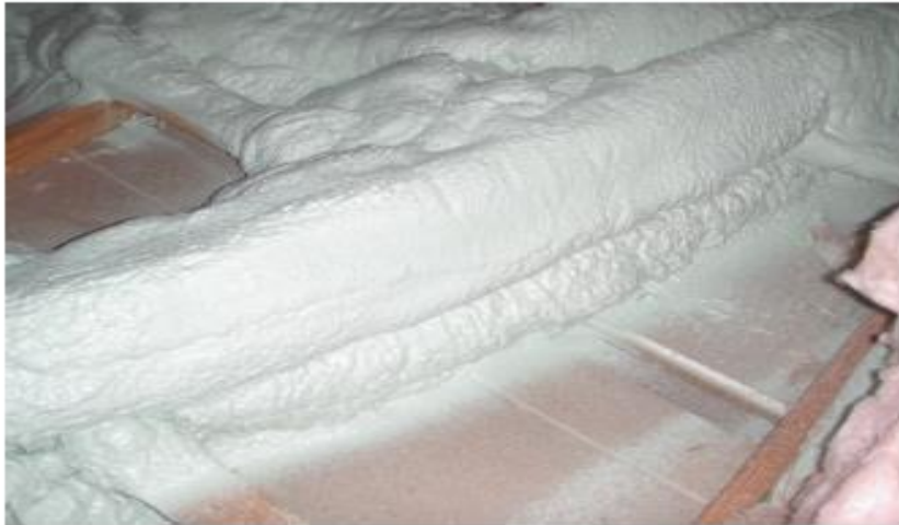
Figure 20. Ductwork well-sealed to sheetrock with ccSPF
