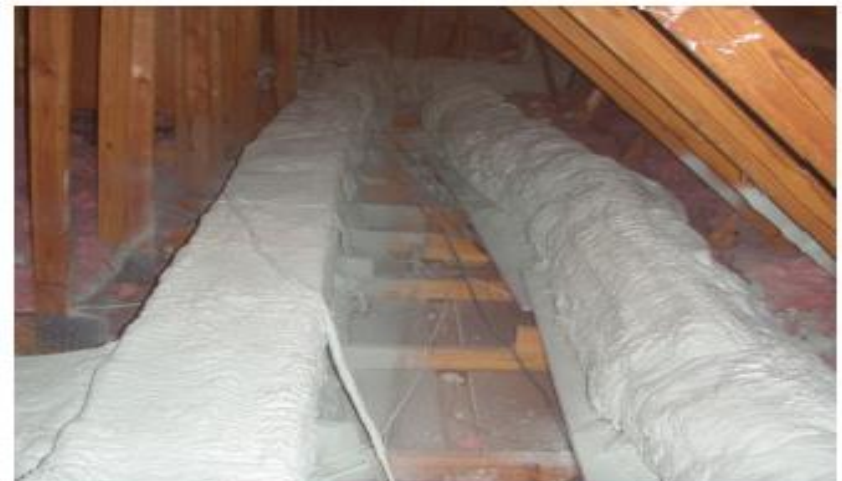
Figure 23. Varying application thicknesses shown on rectangular (left) and round (right) ducts
