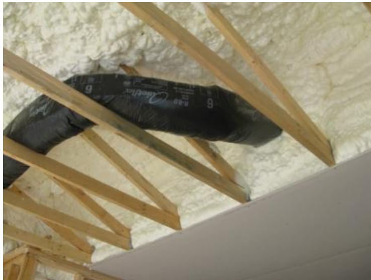
Ducts in unvented attic
