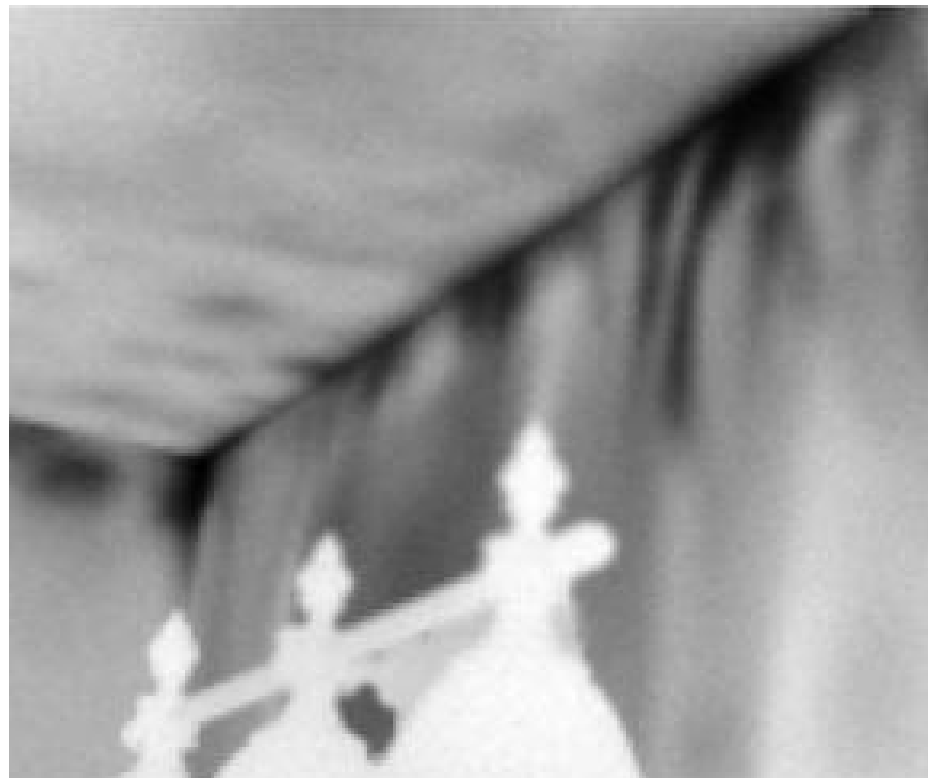
Attic air infiltration into the wall
