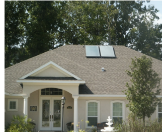
Solar Hot Water
