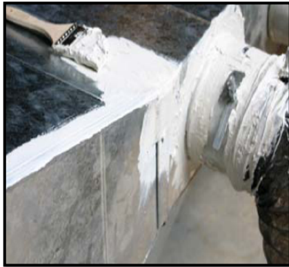
Recommended: Seal all duct connections with mastic
