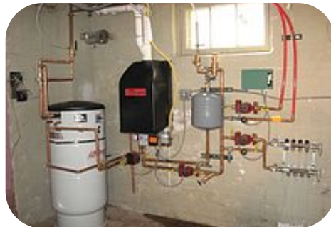
Hot Water Distribution Layout
