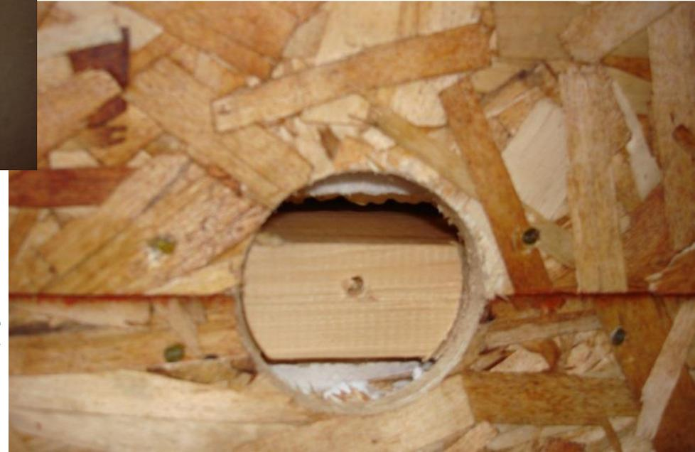
Single spline joint without any seal
