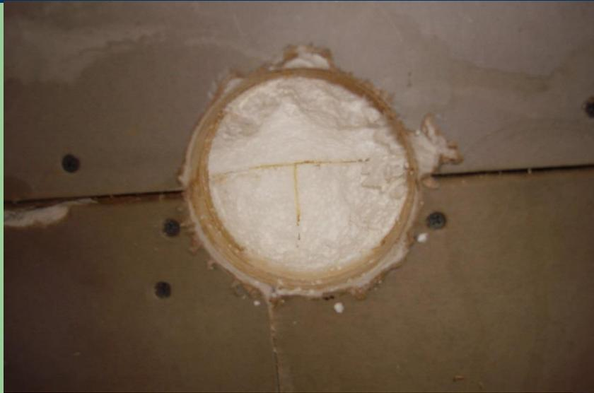
Properly sealed at panel joint
