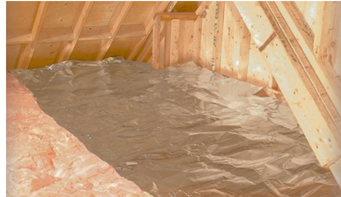
“Horizontal Radiant Barrier” (HRB)
