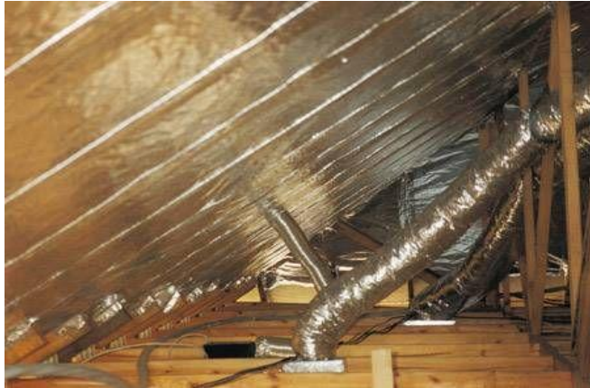
“Truss Radiant Barrier” (TRB)
