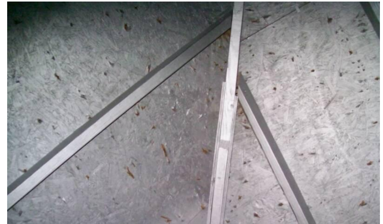
“Interior Radiation Control Coating” (IRCC)
