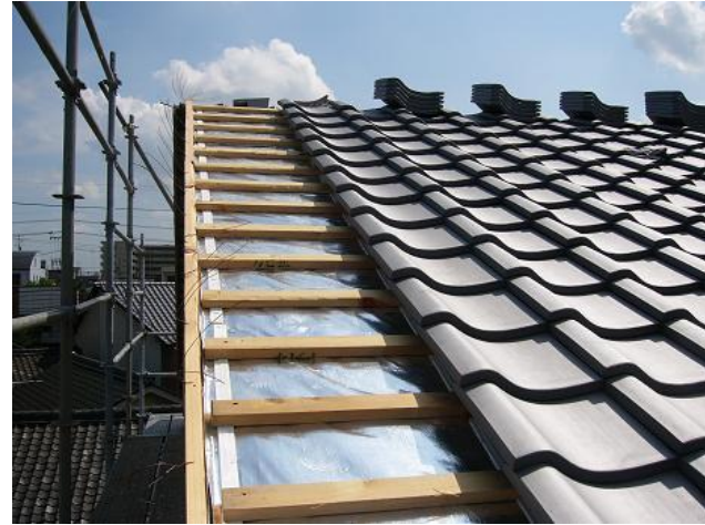
“Radiant Barrier Below Roof Tile”
