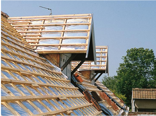
“Radiant Barrier Below Roof Tile”
