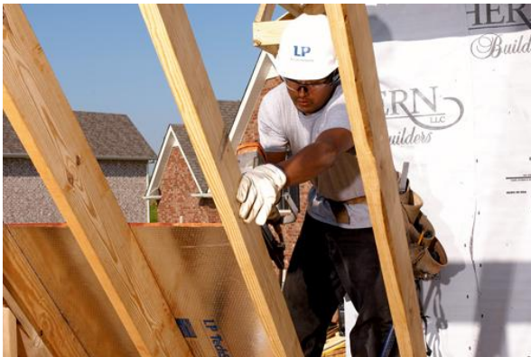
“Deck Applied Radiant Barrier” (DARB)
